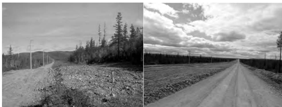
Fig. 6. ESPO sections with an organized technological highway along the pipeline in the conditions of continuous distribution of permafrost. Photo by S.I. Serikov.
